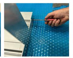
**4.** Decide what end you want the gearbox winder to be installed. Lay out all parts and note the slotted coupling required for handle operation is to be at the top.
